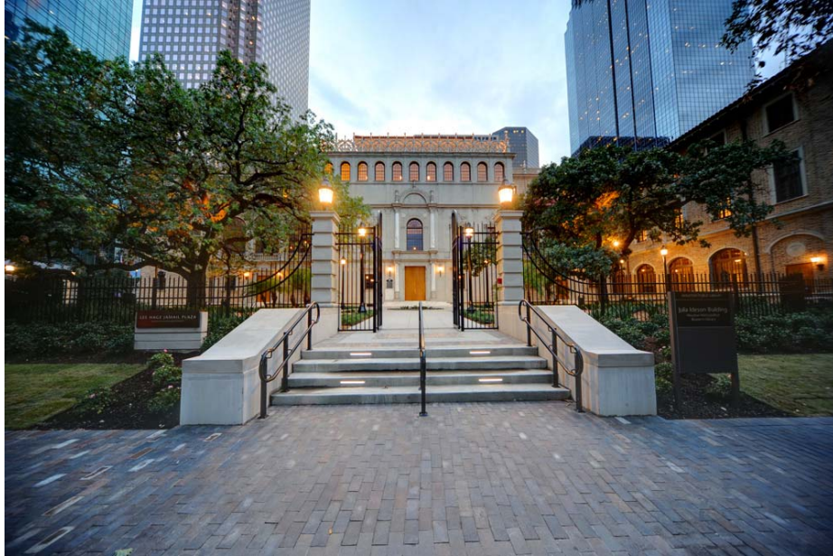
McKinney Entrance to the Julia Ideson Building
